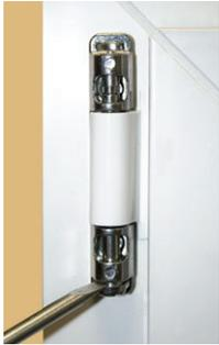
Mount the window handle onto the sash and screw it down. After this, unhook the sash by pulling out the pincer hinge pen until the spring engages. Now open the sash and lift it out.
